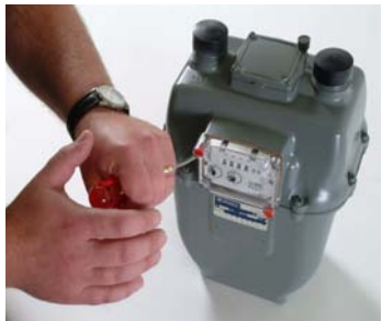
Figure 1 Removing Existing Tamper Plugs
